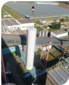
Assembly of a silo for activated charcoal
